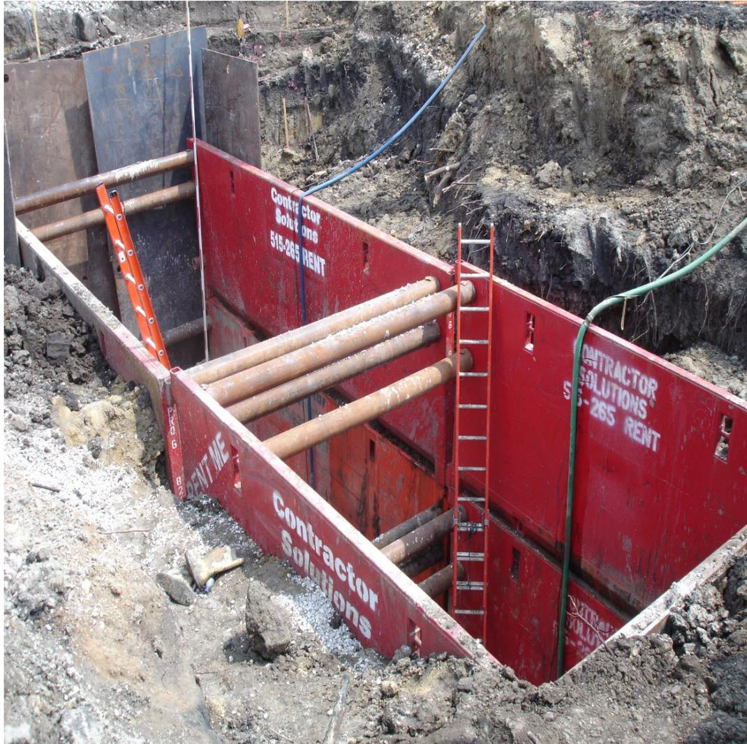
A trench box system will be used to complete the sections of deep sanitary sewer installation to mitigate health and safety risks during construction. One of the benefits of using this method is the reduced excavation footprint.
