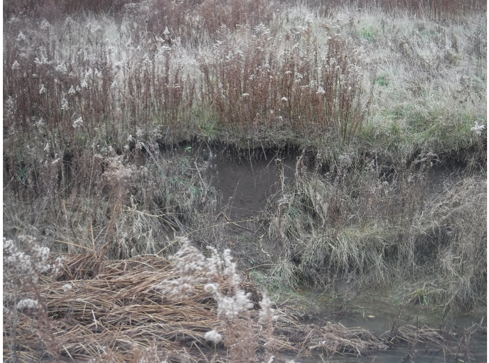
Photo 8: Typical evidence of recent bank erosion along Talbot Creek within the Study Area (facing east).
